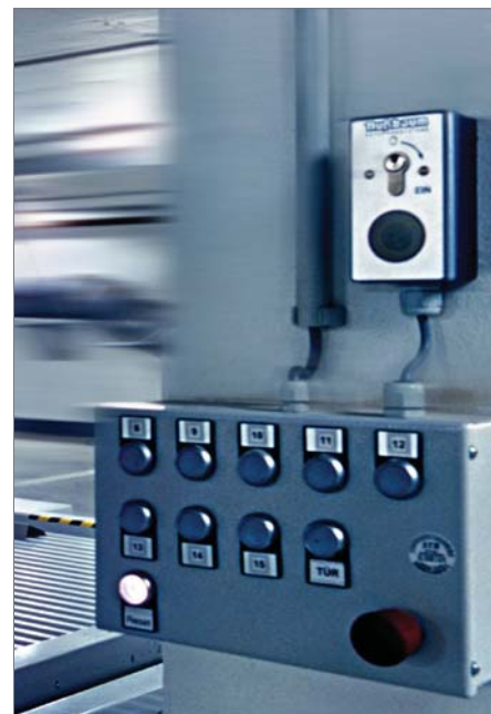
fi g. above: operating panel with dead man's control (freely programmable execution)
